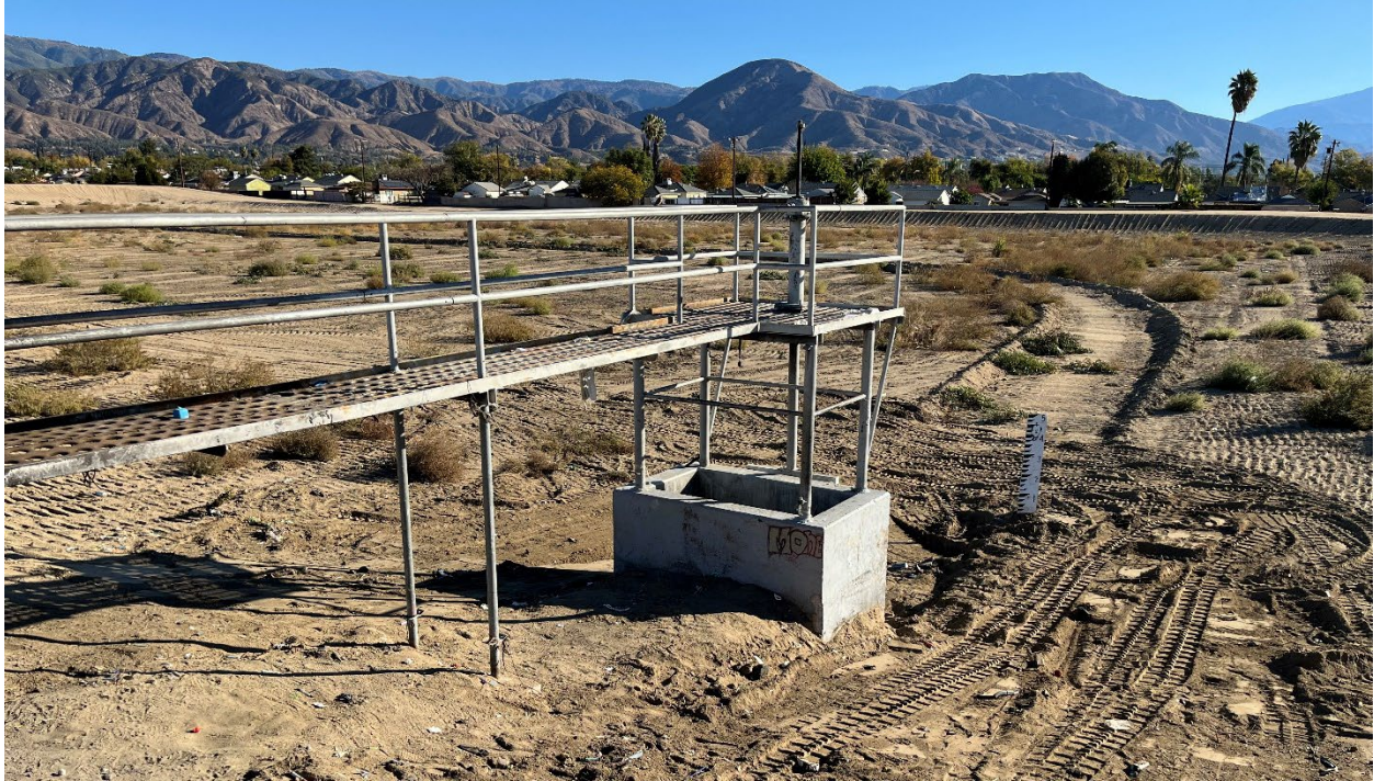
Figure W - Lynwood Basin No. 4 Drop Inlet and Man walk to Slidegate Mechanism
