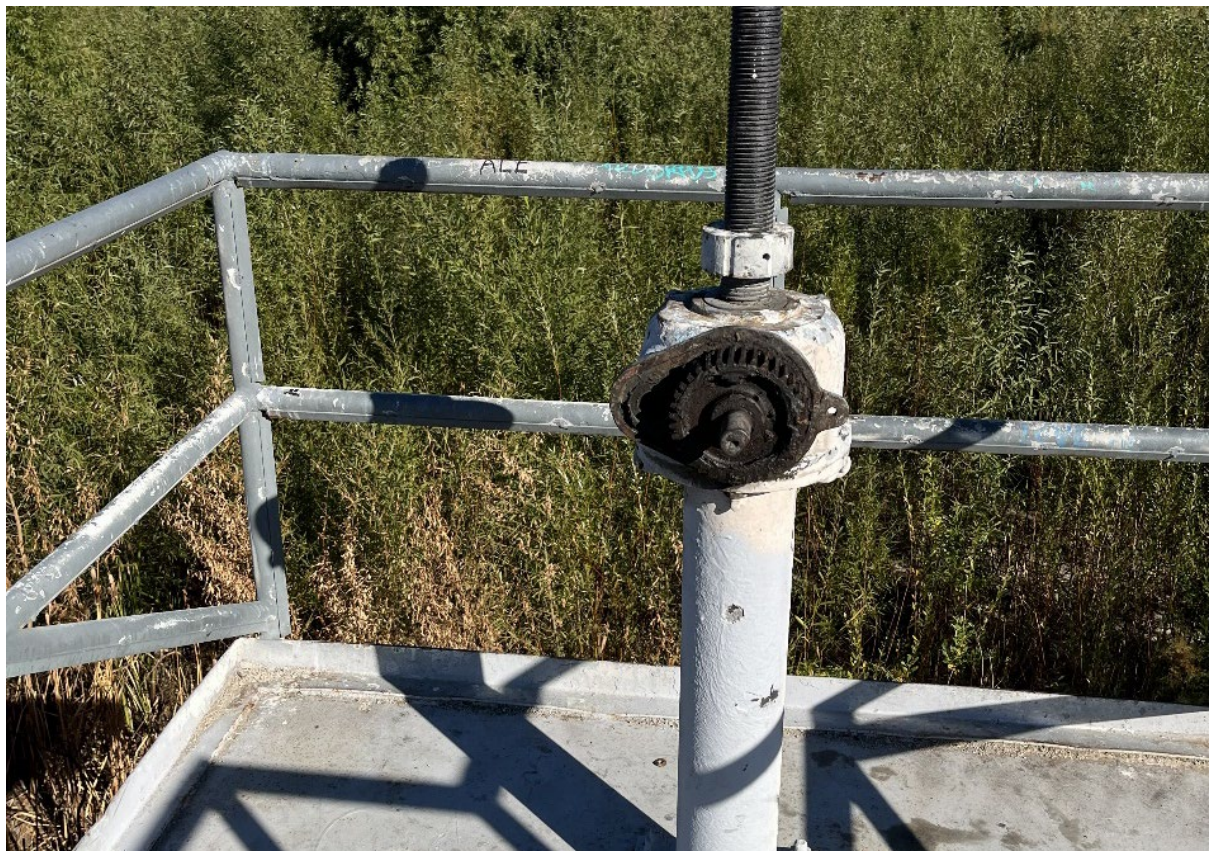
Figure S - Twin Creek Recharge Basins Drain-Gate Mechanism
