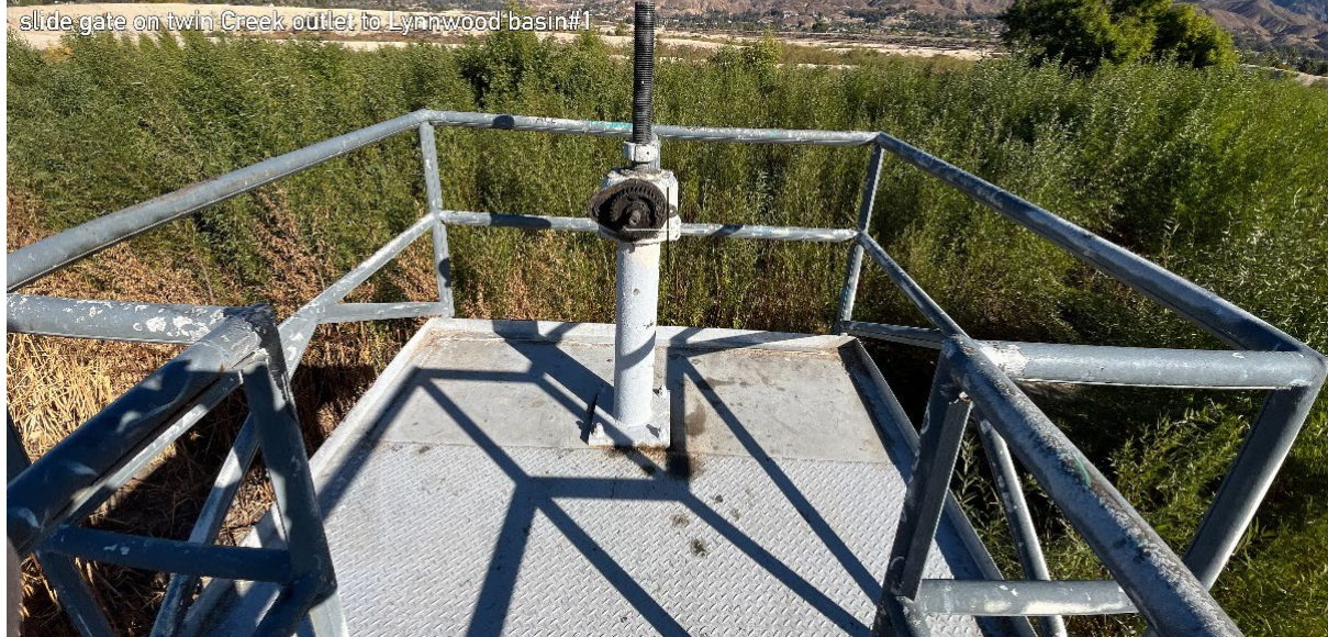
Figure S - Twin Creek Recharge Basins Drain-Gate Mechanism
