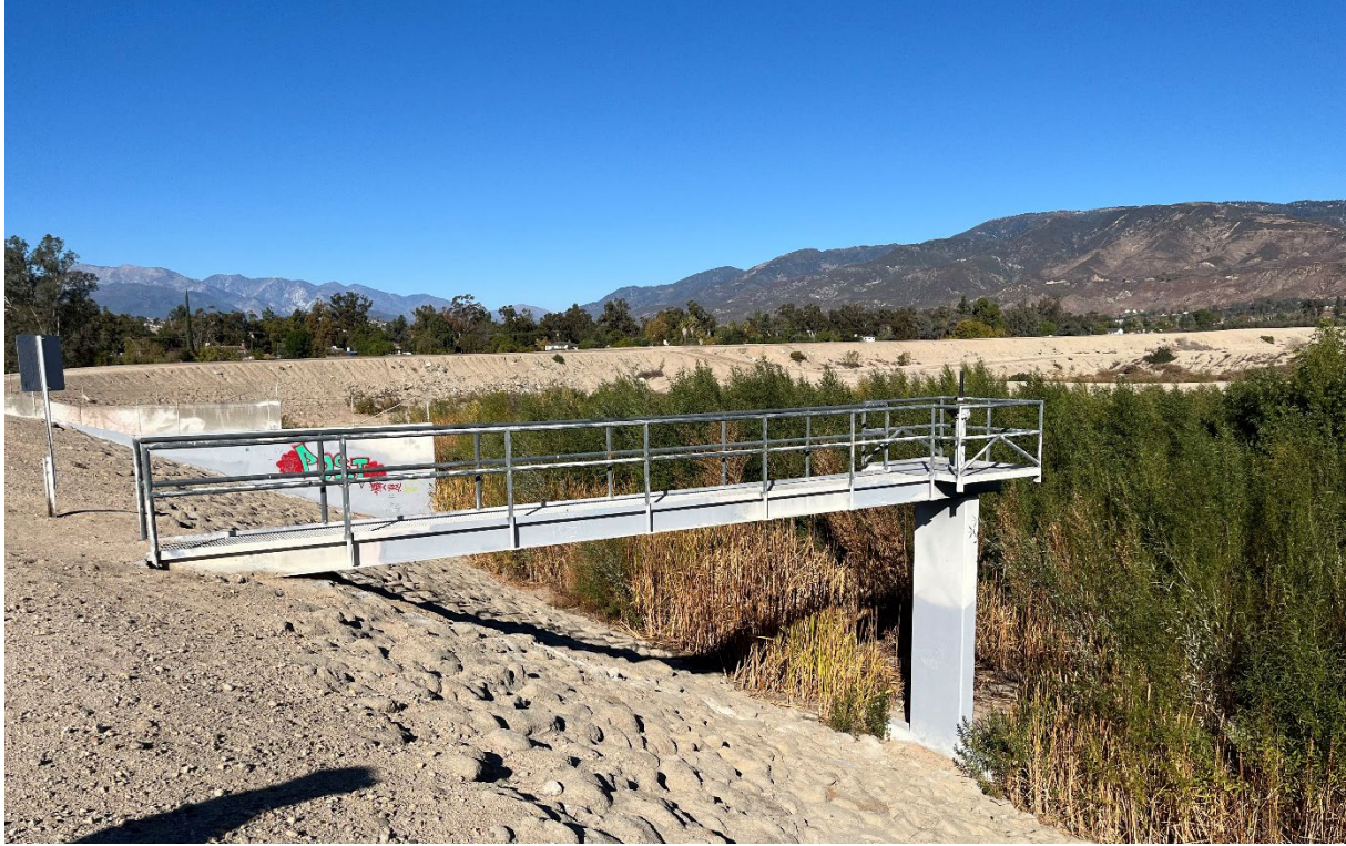
Figure Q - View of Manwalk to Twin Creek Recharge Basins Drain Gate
