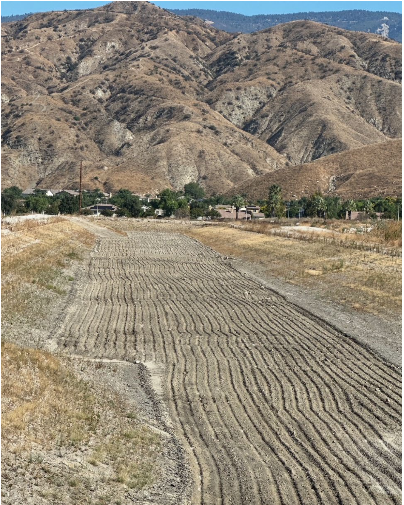
Cleaned SAR Basin 22 on September 29
