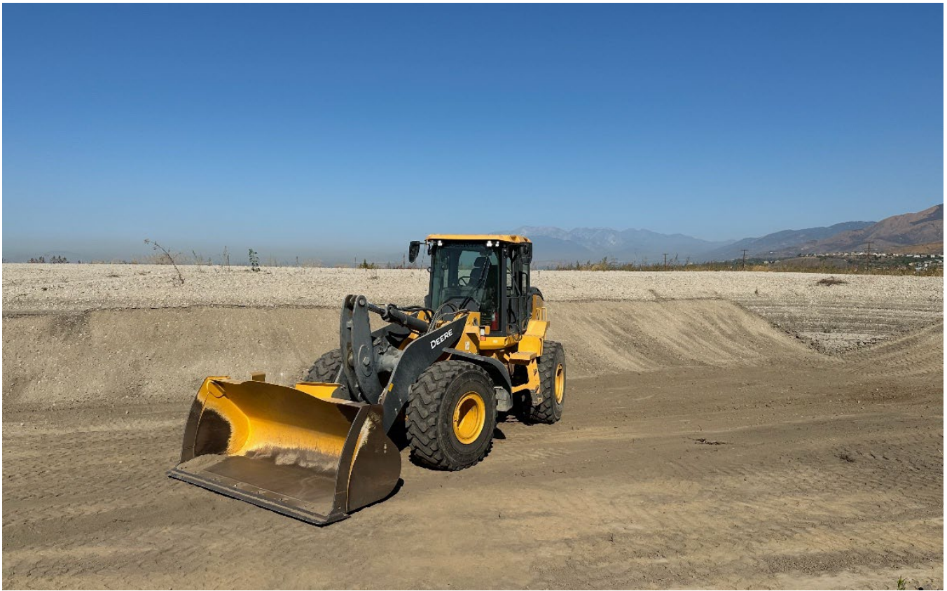
Rented loader used to clean SAR basins 20-22 and 24
