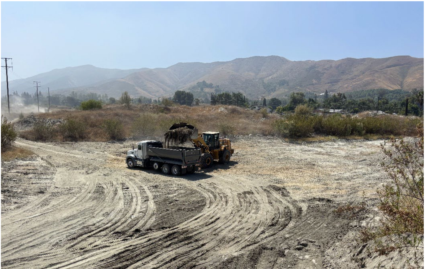
Removal of materials stockpiled during recent basin maintenance on June 20
