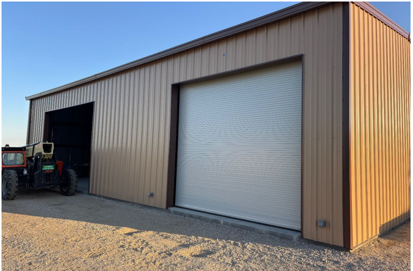
Mentone Shop construction progress
