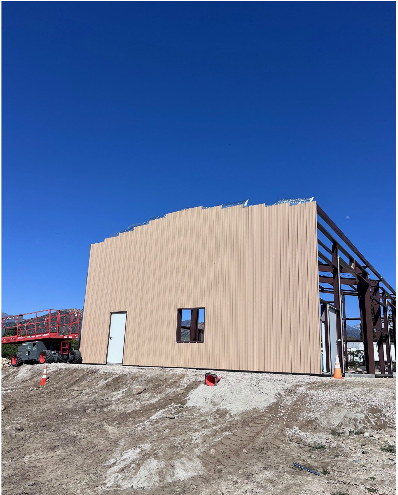
Walls going up on the Mentone Shop on April 7
