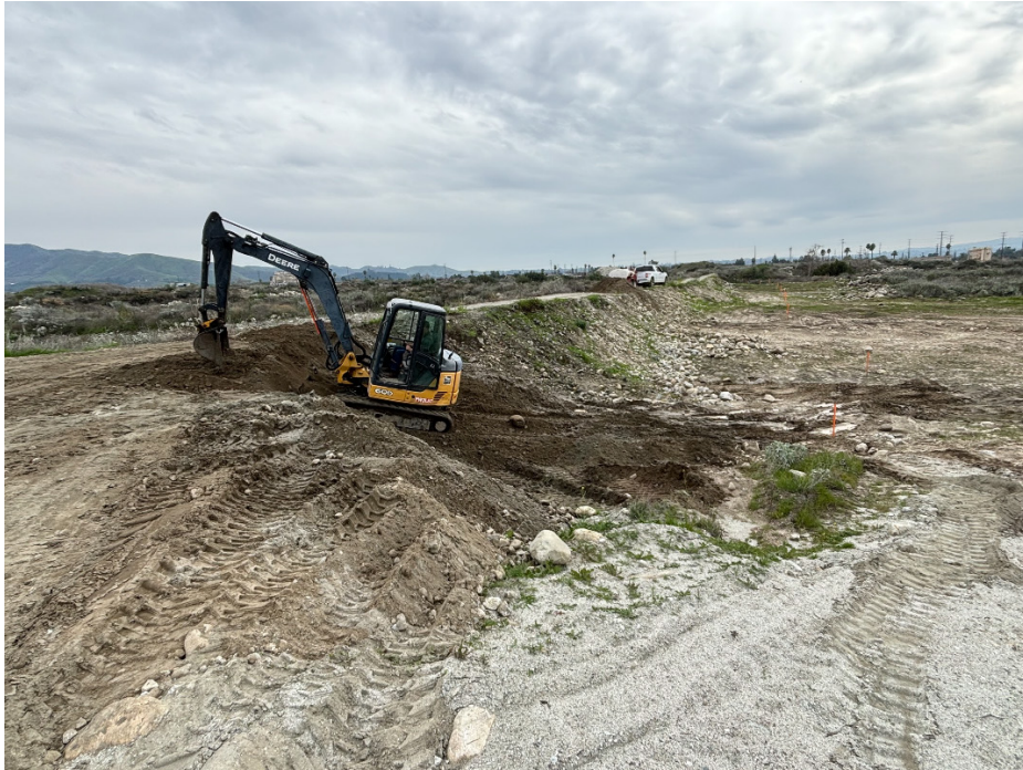
District staff repairing roads and berms before a storm
