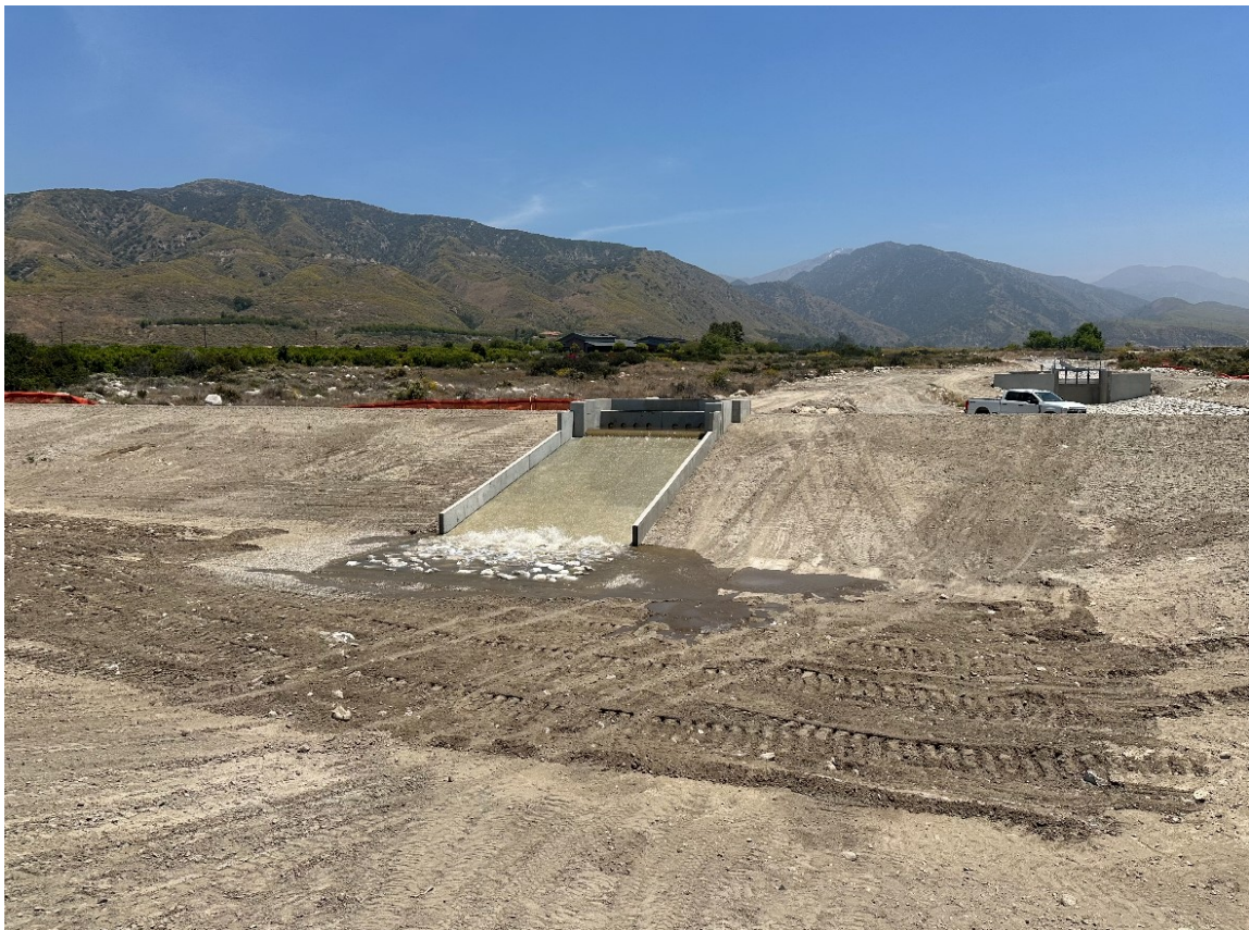
The first recharge water entering Enhanced Recharge Basin C on June 4
