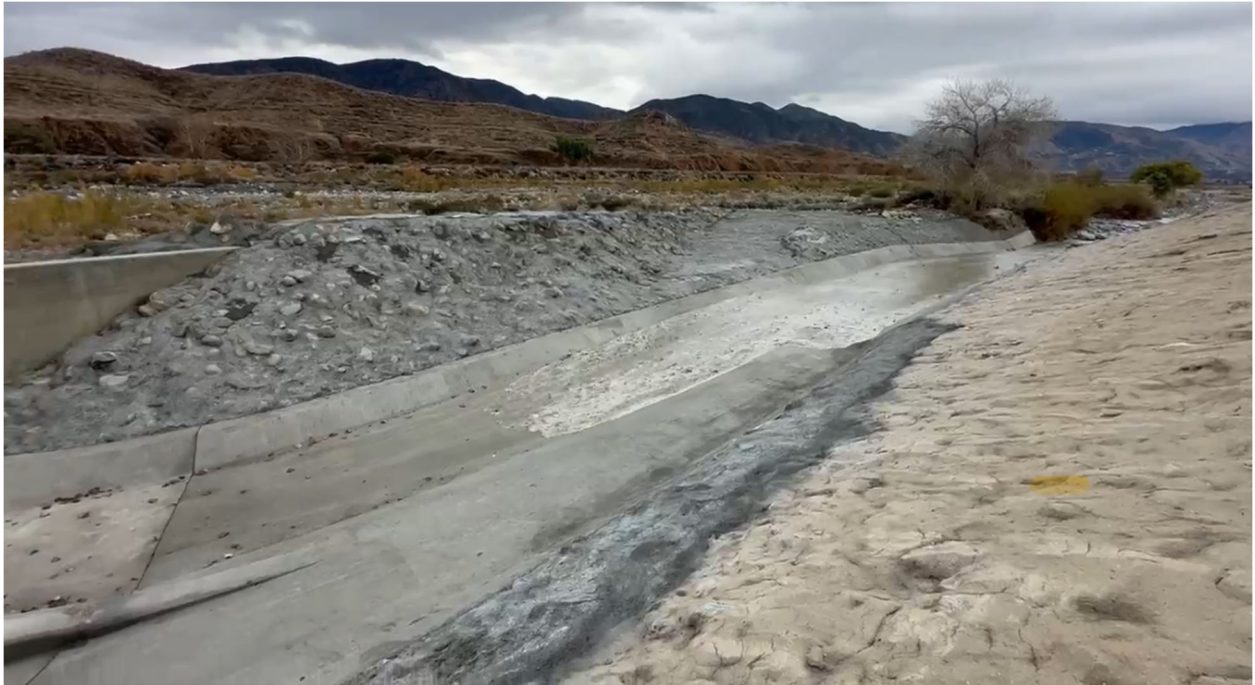
First flows entering the new Mill Creek Diversion
