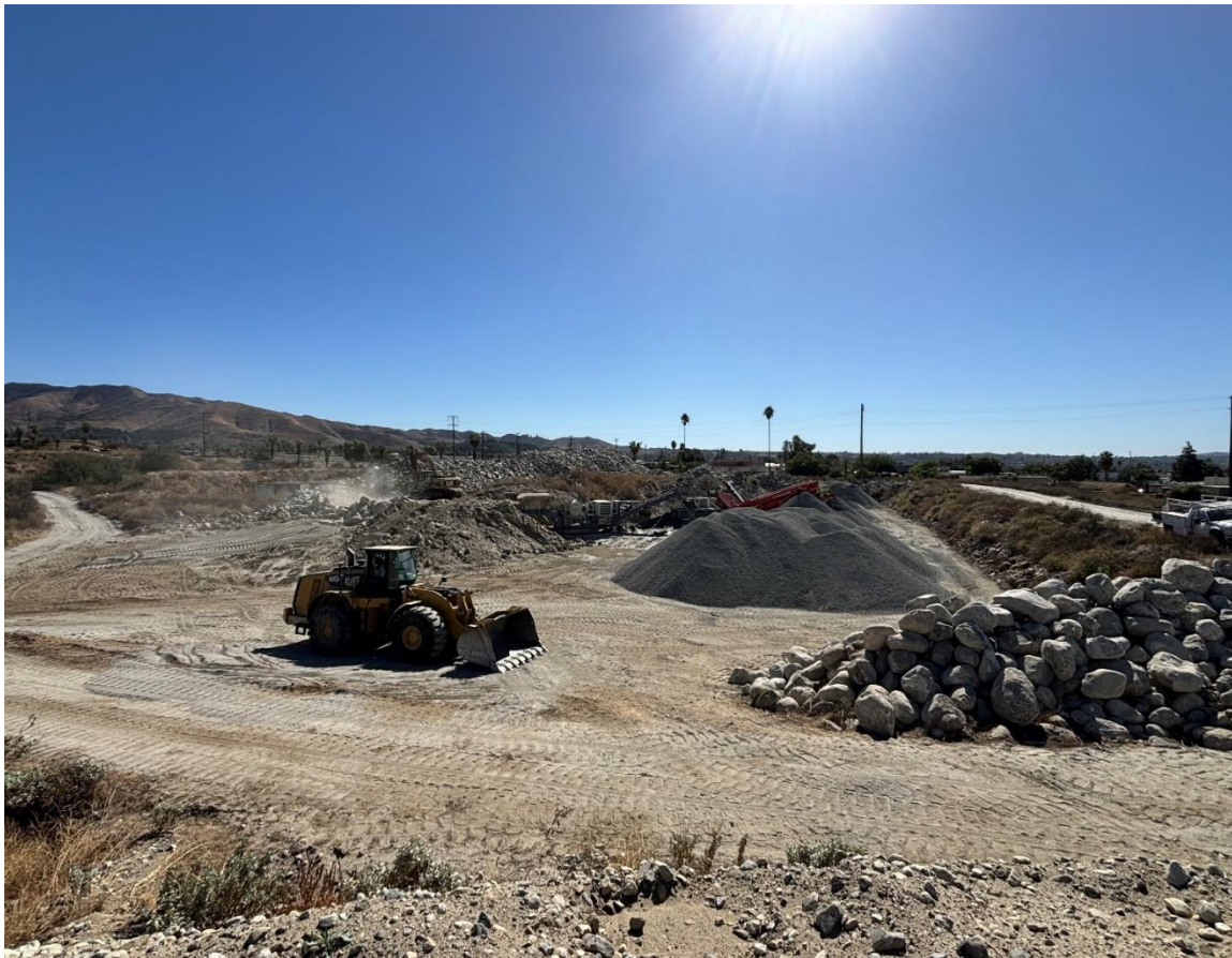
Continuing Stockpile Processing at Mill Creek Pond 24 on November 5
