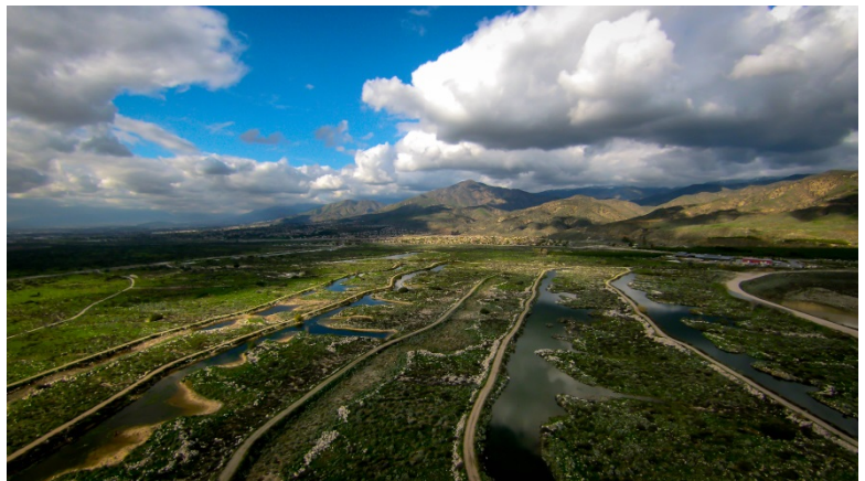
District Percolation Basins
