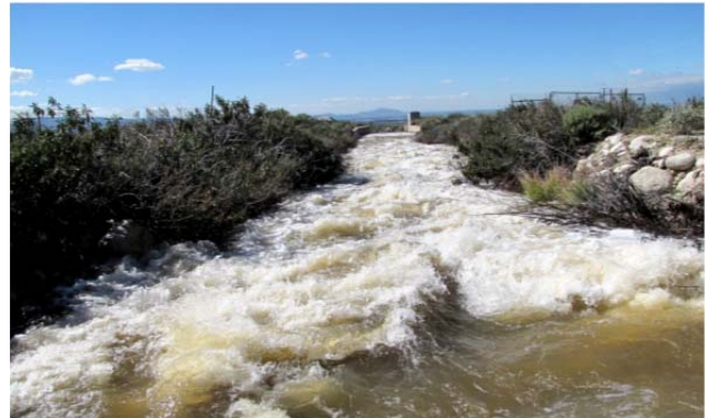
District Main Canal to Santa Ana Basins
