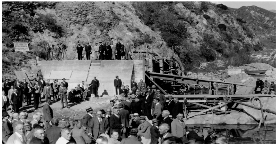
Cuttle Weir Diversion Structure Dedication
