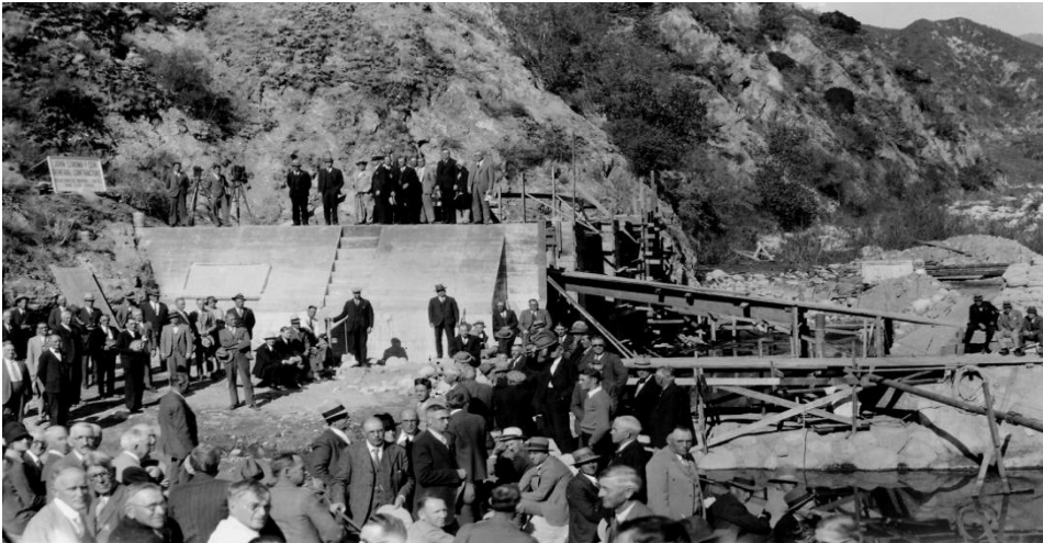
Cuttle Weir Diversion Structure Dedication
