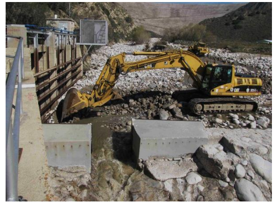
Diversion Maintenance Activities
