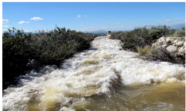
District Main Canal to Santa Ana Basins
