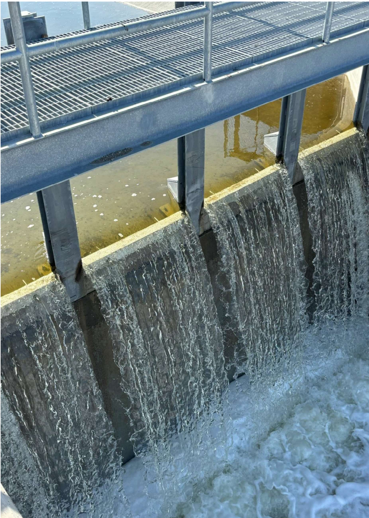
Water flowing into the canal upgraded by the Enhanced Recharge project on August 8
