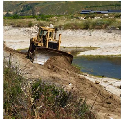
Basin Maintenance Activities
