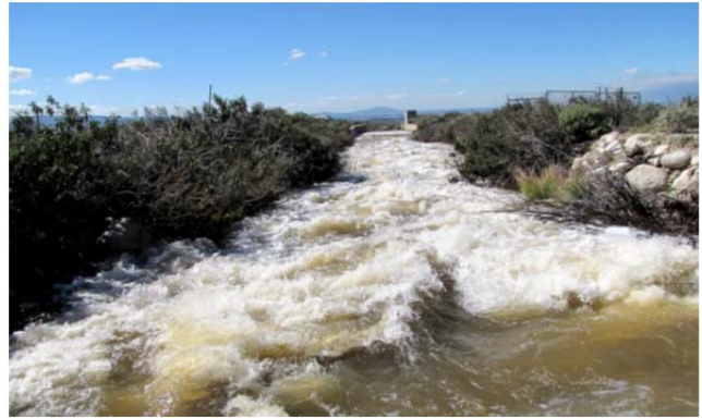
District Main Canal to Santa Ana Basins
