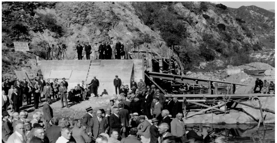
Cuttle Weir Diversion Structure Dedication
